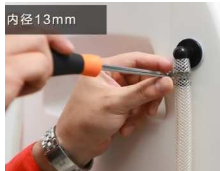
Fixing the Drain/ Overflow Lines
